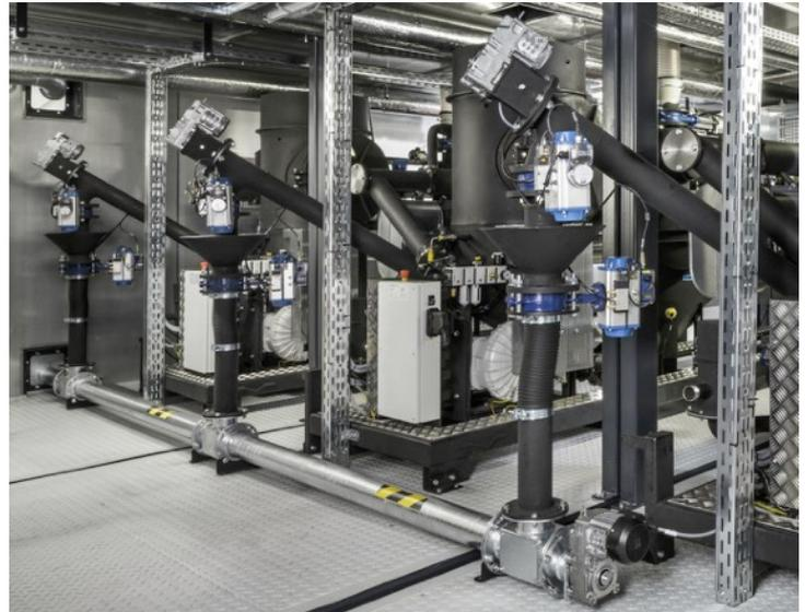
Sunnytek & Partners are happy to offer this total energy solution based on wood gasifier and a gas engine with an electric generator. The system is fully automatic and use wood chips and biomass to produce electricity and hot water. Total efficiency is over 90%.
