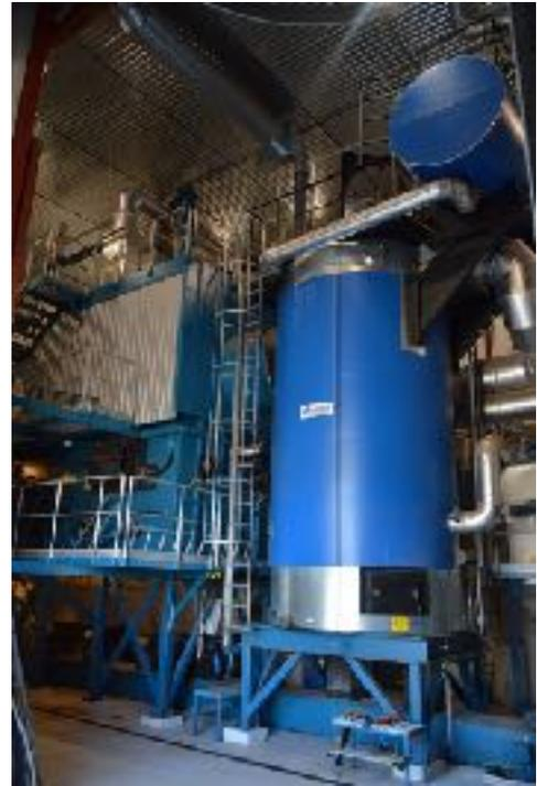
Tubes with the very efficient Rockwool insulation systems that save heat inside boiler and not in the boiler room
