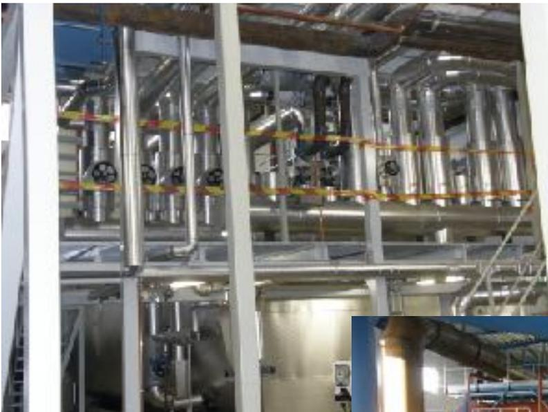
Boiler room for a large 16 MW boiler in Ekenäs. This have a water jacket boiler room and plenty of tube sto collect all heat.
