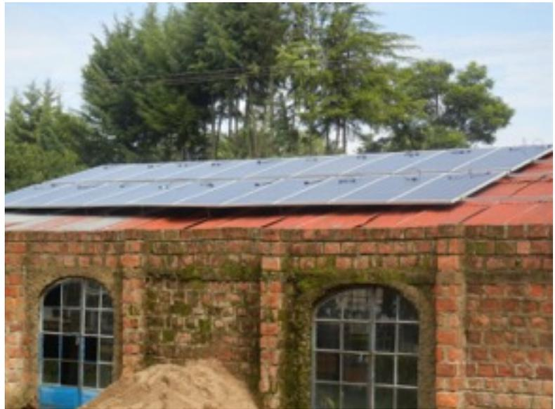
**Dormitory system in school Kenya** 2014 we installed about 25KW solar panels and a battery system of almost 100KWH in Kericho in Kenya. System handle a dormitory of 700 students with 100% of energy needs. We use 250 W solar panels combined with the 931 AH OPZV battery by North Star. Photo show 1 set up of panels of 12.5 KW and battery back up system. Inverters are 3 Phase 2X12 KW output with MPPT chargers.
